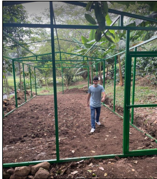
Esteban in the nearly finished greenhouse!
